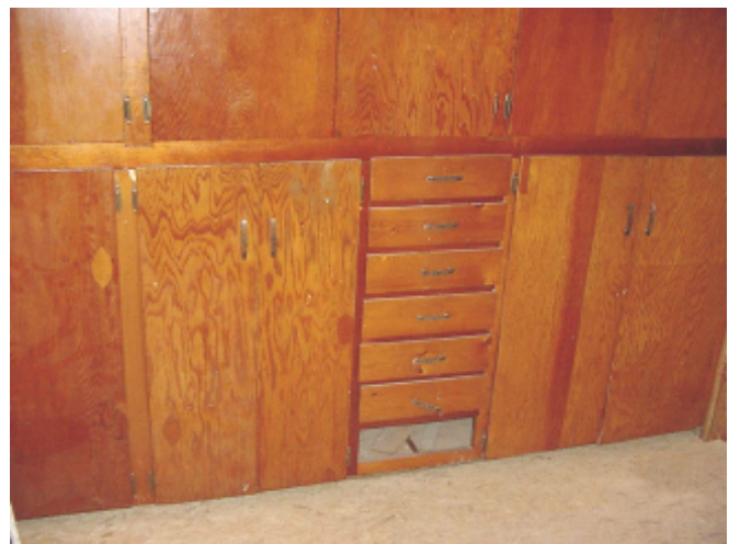
FIGURE 15.10 Surfaces that may have had paint stripped.
