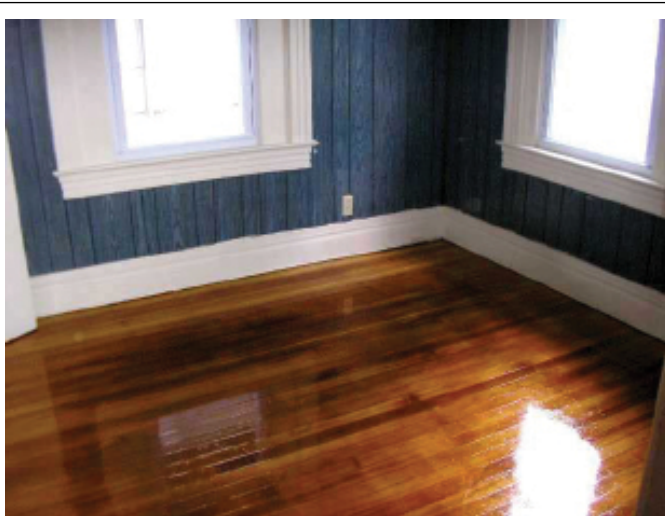
FIGURE 15.6 A floor that may be tested.
